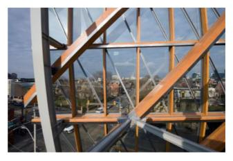
In front of the arch layer lies the rectilinear glulam mullion grid that is linked back to the glulam arches using stainless steel connecting rods with pivoting ball joint connections. The mullion grid curves over and around the arches and is allowed to move within its own plane relative to the glulam arches to accommodate relative movement. The glazing system is mounted to the face of the glulam mullion grid.
